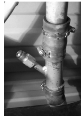
Figure 7: Installing 'Return To Tank' assembly
